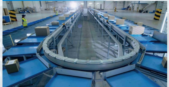
Logistics conveyor line
